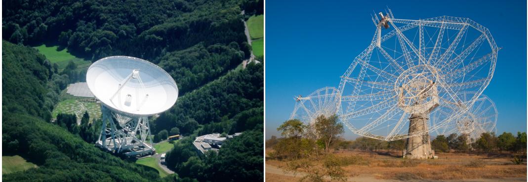
Figure 7.15: Left : the 100 metre Effelsberg radio telescope in Germany. It is the world's largest fully steerable single-dish radio telescope. Right : three of the 30 total 45 metre dish telescopes of the Giant Metre-wave Radio Telescope (GMRT) interferometer in India. Image credit: dr.G.Schmitz (Effelsberg); NCRA-TIFR (GMRT).
